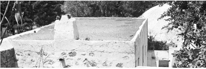
Fig 16. Soil rooftop of a typical Bodrum House (photograph by H. Tanrıöver, Bodrum 1967)
