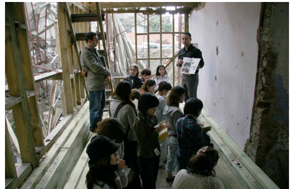
Site visit to an ongoing restoration by KUDEB
