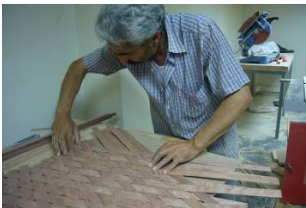
The wickerwork ceiling
