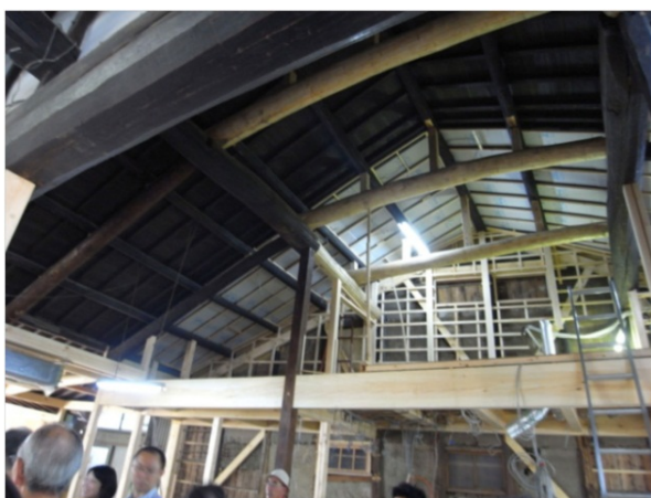
Fig.3) Refurbishment of Kyo-machiya . Some members of framework are partly replaced.
