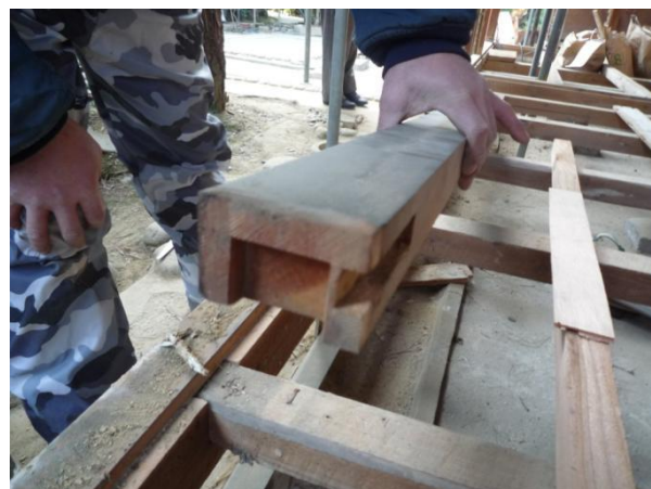
Fig.4) Dismantlement and reconstruction in a new site; connection of the threshold sill.
