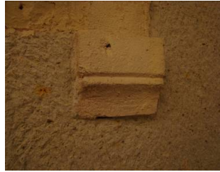
Fig. 33 Stone combination detail at a rock-cut wall
