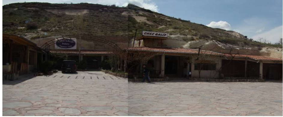
Fig. 36 The lean-to roof added to the entrance by the owner
