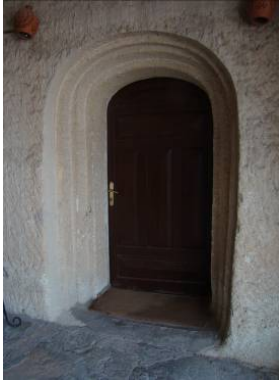
Fig. 35 Service Entrance Door
