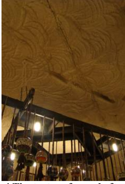
Fig. 4 The texture formed after the extraction of big rock masses via machines
