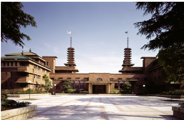
Fig. 1. The Koshien Hotel (presently Koshien Kaikan)
