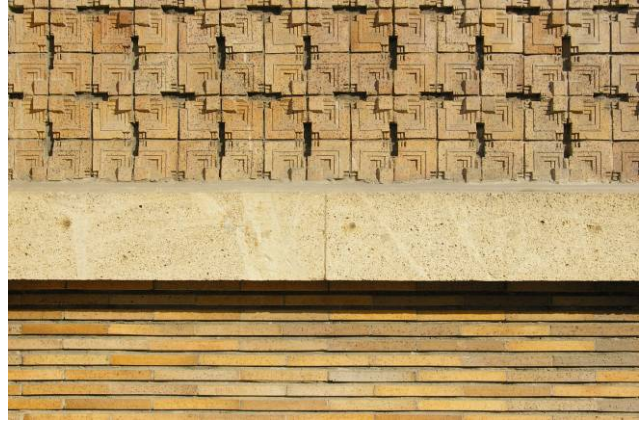
Fig. 12. Square tiles (above), border tiles (below)
