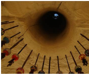
Fig. 23 Natural ventilation tunnel
