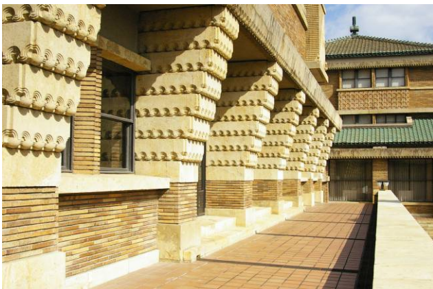
Fig. 11. Columns with a span of two 'ken'
