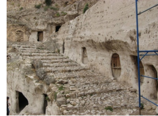
Fig 31. Settlement Where Carving Utilized as the Fundamental Building Production Method-Hasankeyf
