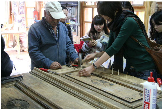
Working at the bottega: Students as working on the repair of worm holes on the door from 200 years ago
