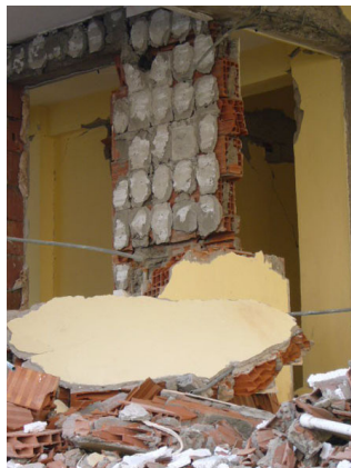
Left: This type of ceramic block is used everywhere. We had never witnessed that the wall of concrete being housed in the frame of RC structure under construction.
