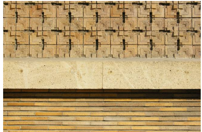
Fig. 12. Square tiles (above), border tiles (below)
