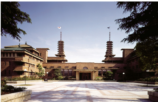
Fig. 1. The Koshien Hotel (presently Koshien Kaikan)
