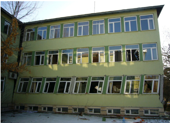
Left: We returned from Erciş city to Van city, and inspected damaged Waterworks Bureau building. There was no wall on the first floor of the extended annex buildings. The building has lost connections at the L-shaped corner.
