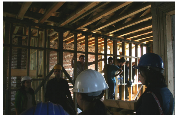
Wooden structure being refurbished, the hall on the second floor
