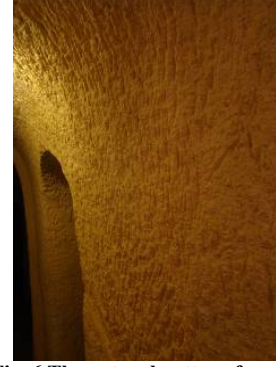
Fig. 6 The natural pattern formed due to hammer marks on walls done by hand workmanship
