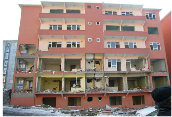
Right: A leaning collective housing on the brink of collapse. We were told since the building was built on the basis of a dry riverbed the damage had been that much larger.
