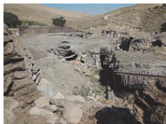
Fig 27. Collapsed house in Besler Settlement.
