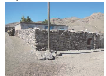
Fig 25. House with a courtyard enclosed with stone walls in Besler Settlement. The walls secured height to make it difficult to be looked in.
