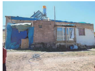
Fig 19. Brick house in Konaklı Settlement.
