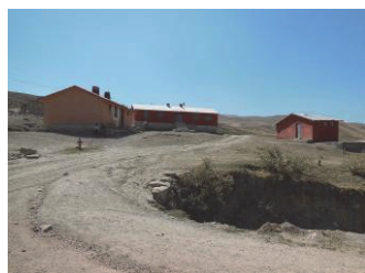
Fig 31. Primary school on west outside of Besler Settlement.
