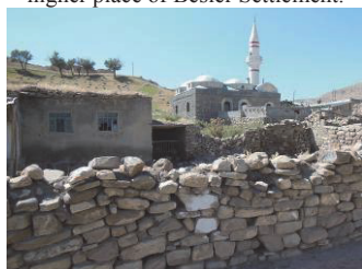
Fig 32. House and livestock barn integrated with walled courtyard in Besler Settlement. Mosque behind had small domes, minaret and different shaped windows from the other houses in settlement.
