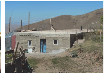
Fig 20. Concrete house in Konaklı Settlement.
