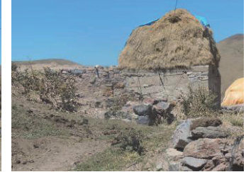
Fig 12. Haystack on flat roof of building in Konaklı Settlement.
