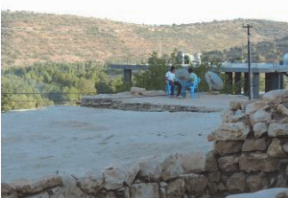
Fig 34. Rooftop used as terrace in Aran Settlement.
