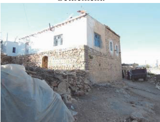
Fig 32. Upper floor partly extended or reconstructed and painted white in Aran Settlement.
