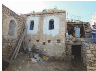
Fig 29. Traditional house, whose semi-underground first floor was used for livestock in Aran Settlement.
