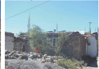
Fig 14. Stone house in Konaklı Settlement.
