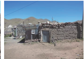
Fig 16. Houses and livestock barns sharing walls in Konaklı Settlement.
