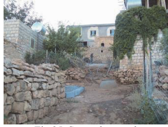
Fig 25. Steep slope path perpendicular to contours in Aran Settlement.
