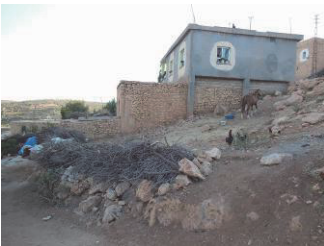
Fig 30. Concrete extensions or reconstructions to upper floor in Aran Settlement.
