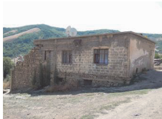
Fig 16. Houses with downstairs partly under slope in Çevre Settlement.
