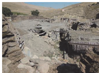
Fig 27. Collapsed house in Besler Settlement.
