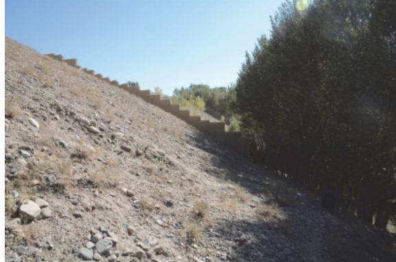
Left: Point 70, South view of the west terrace. Right: Point 74, Retaining wall on the south boundary of the planned area. Retaining walls are made by adobes.
