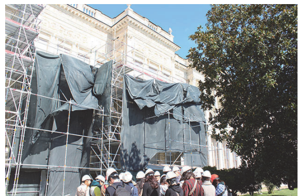
Visiting the restoration site of the building for crown prince
