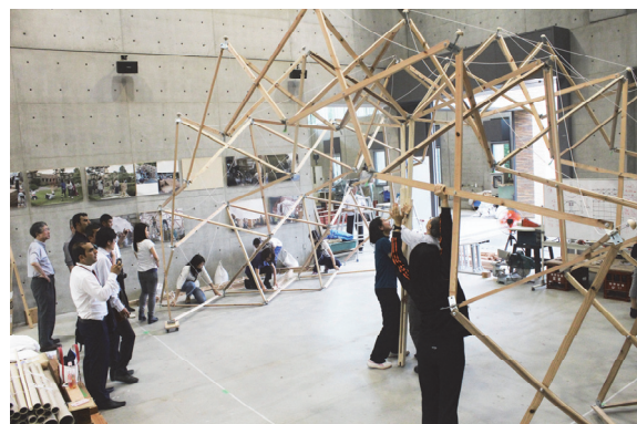
Visit to Department of Architecture and Architecture Major: vault space by the scissors construction method
