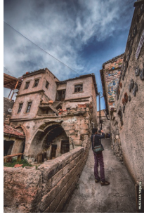
Photograph 3. Avanos Traditional Rock Civil Architecture Examples (Taşkın, M., 2016)
