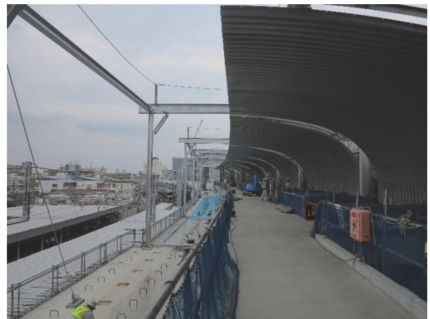
Figure 27. View east of platform
