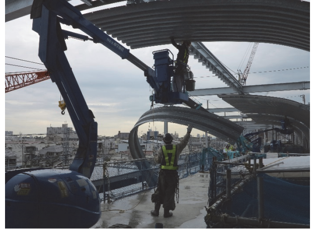
Figure 26. Set-up of plank sheets
