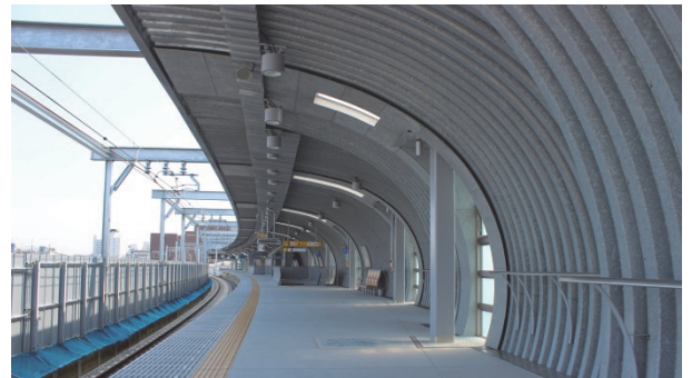
Figure 16. View east of platform
