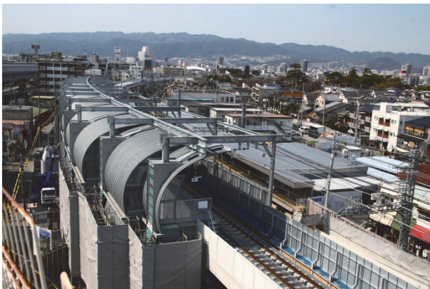
Figure 1. Birds-eye view of Hanshin Electric Railway Naruo Station
