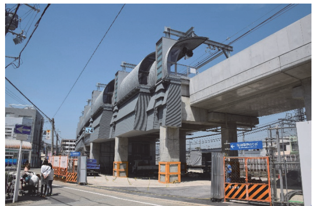
Figure 3. View of east end of platform from southeast side
