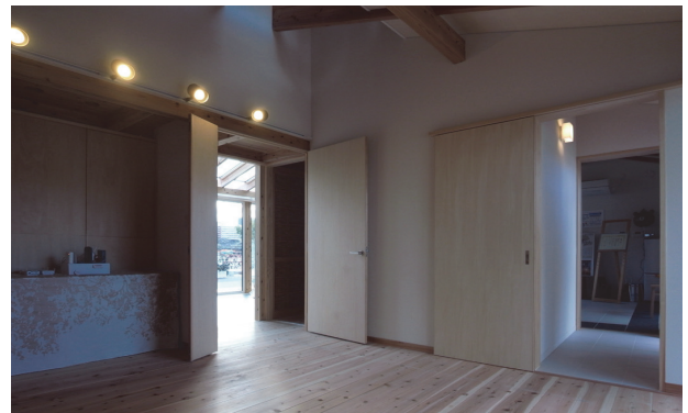
Figure 5 Inside the kura space: the space is isolated from the surrounding room by highly insulated partitions to create a private living space with a stable temperature.
