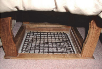
Figure 6. Hori-gotatsu is a “trap” on the heat pit to protect from fire. The temperature of the fire is protected by the ash placed on the trap. ( http://www.daveahlman.net/Old_site/daveinjapan/arch/arch.htm )
