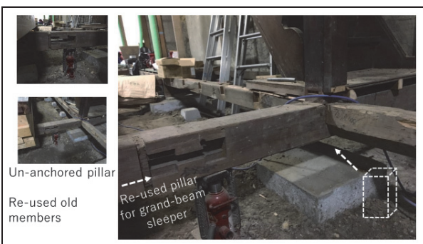
Figure 22: Re-used pillar for grand-beam sleeper.
