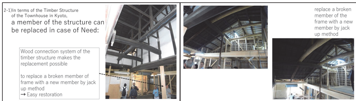
Figure 20: A member of the timber structure in kyomachiya can be replaced in case of need.
