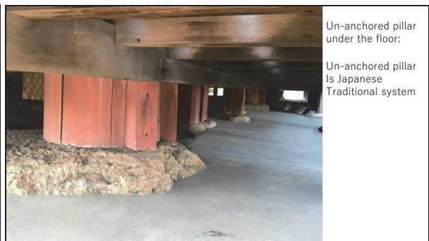
Figure 12: Japanese traditional structure system: Un-anchored pillar under the floor.
