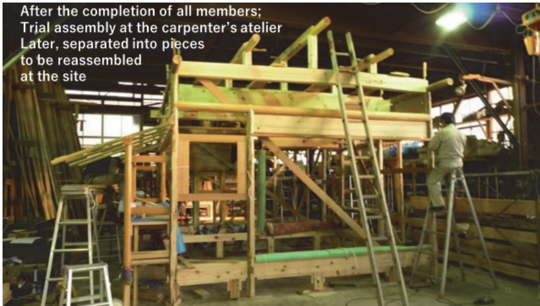
Figure 36: Trial assembly of the traditional teahouse in the carpenter's atelier: Later on, the structure can be separated into pieces to reassemble at the site.
