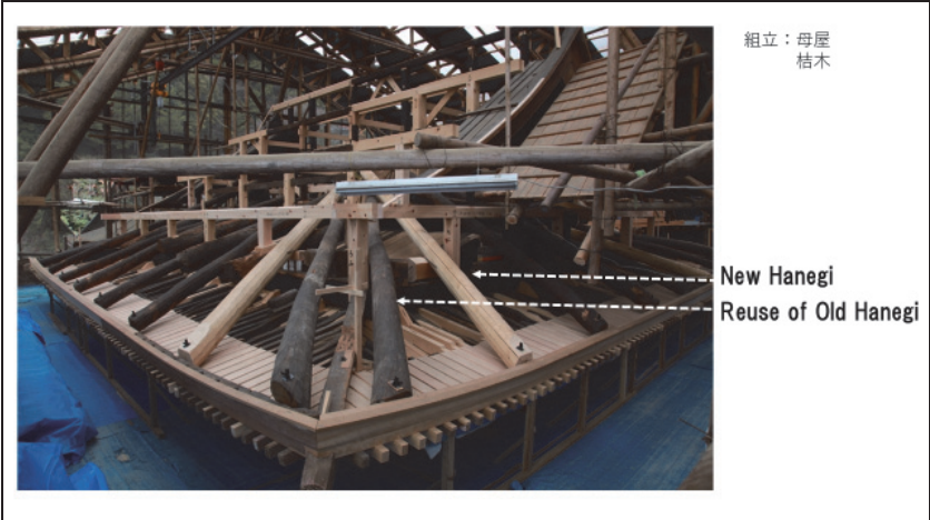
Figure 48: New hanegi and old hanegi reused.
