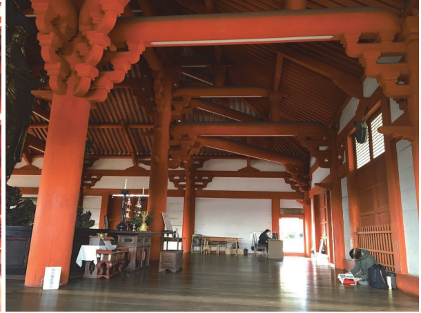
Figure 4: There is no ceiling surface, all the structural members are visible. Composition of three beams and extensive use of tie beams.
