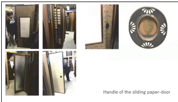
Figure 30: Handle of the sliding paper door.
