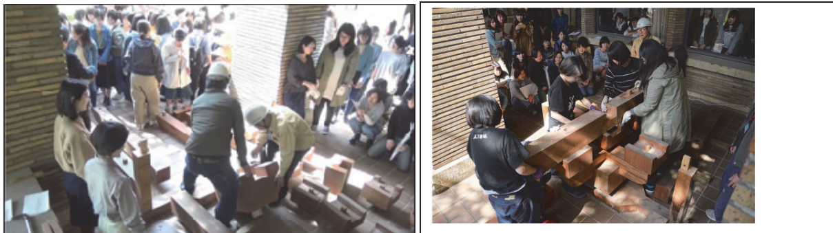
Figure 43: Assemble process of the mockup of square framing of eave of pagoda.
