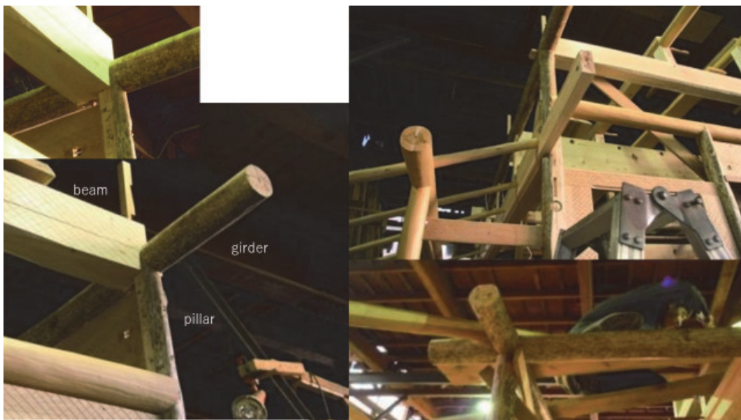
Figure 37: Details of joints.
