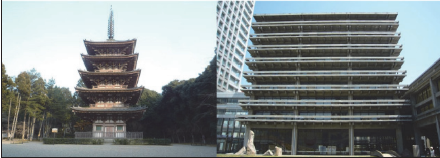
Figure 44: Architect Kenzo Tange attached beautiful eaves to each floor in the design of the Kagawa prefectural office building. It has a high reputation in the worldwide for expressing the traditional space of Japanese architecture with reinforced concrete.
