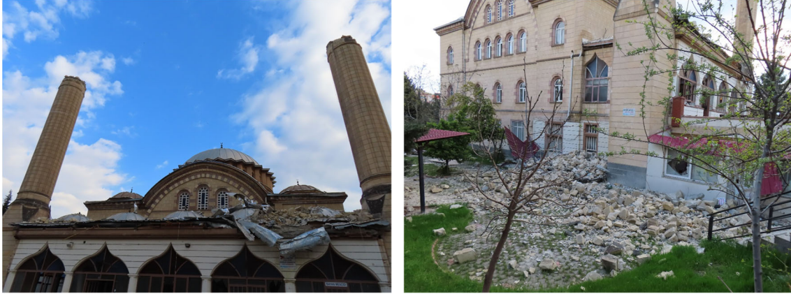
Photo 2-6 Seismic damage in Kahramanmaras (Location ④)
