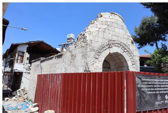
Photo 1-43 Antakya, Hatay. Sarıme Camii
