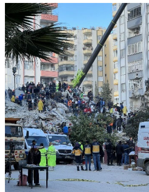
Photo 2-2 Collapse of 14-story apartment
