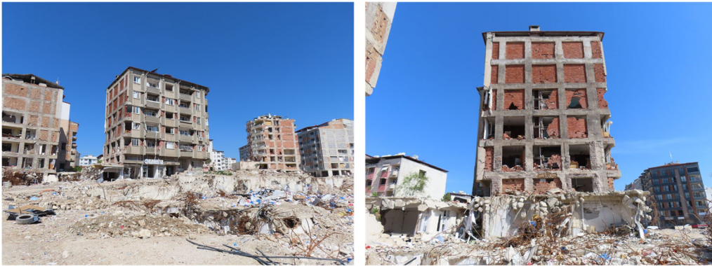
Photo 2-9 Seismic damage in Antakya new urban area
