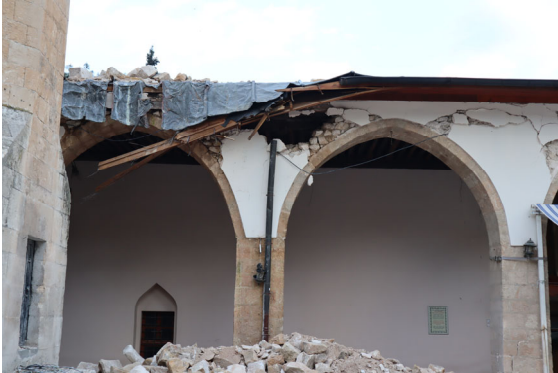
Photo 5-3 Damaged portico.
