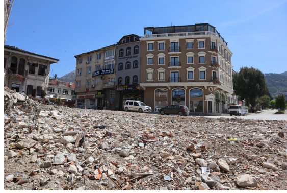
Photo 1-40 Antakya, Hatay. There was also an intact hotel.
