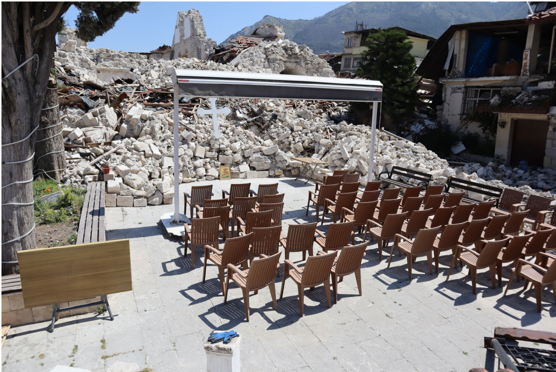
Photo 1-34 Antakya, Hatay. Greek Orthodox Church.
