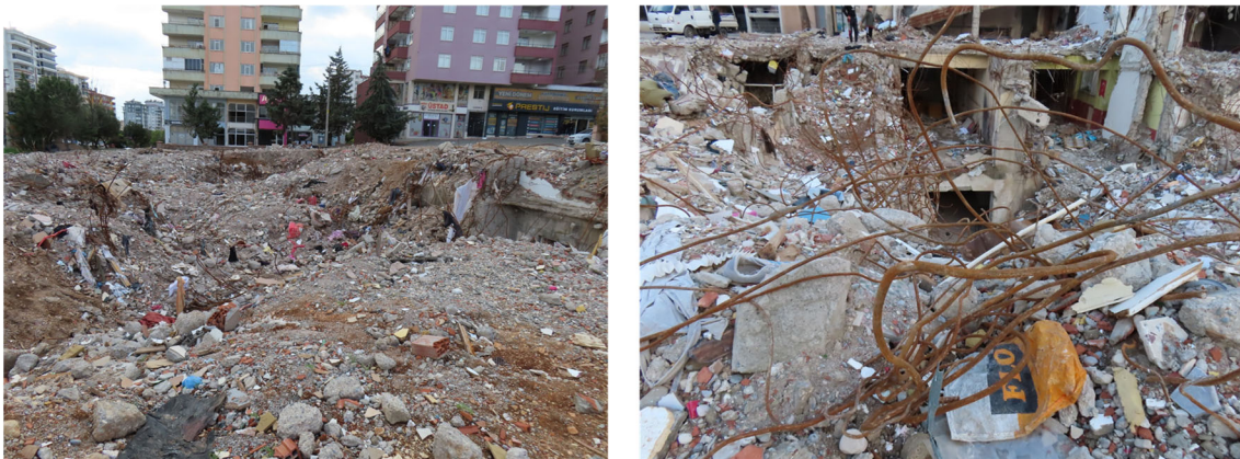
Photo 2-5 Seismic damage in Kahramanmaraş (Location ③)
