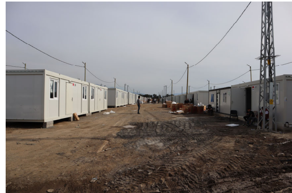
Photo 1-69 Payas, Hatay. Container temporary housing under construction.
