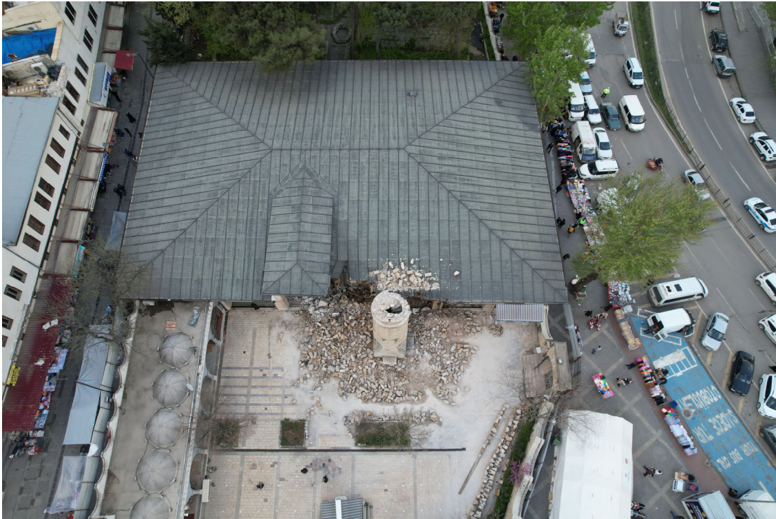
Photo 5-12 The building was damaged by the minaret collapsing and falling stones.
