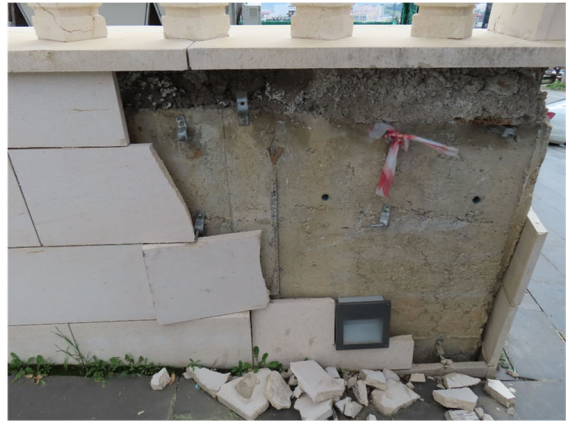
Photo 2-3 Seismic damage in Kahramanmaras (Location ①)
