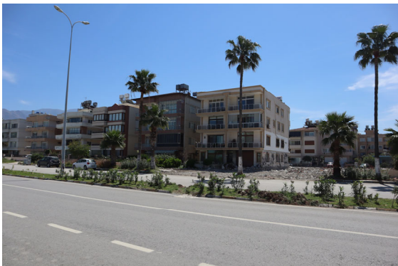
Photo 1-62 İskenderun, Hatay. A 9-story apartment building collapsed. 4-story buildings are safe.
