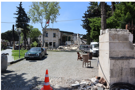
Photo 1-38 Antakya, Hatay. Government building.
