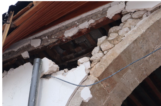
Photo5-6 Arch section of portico
