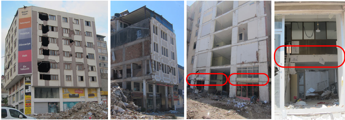
Photo 3-2 Buildings with Commercially Used Lower Levels and Mezzanine Floors
