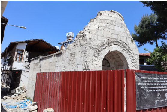
Photo 5-21 Antakya, Hatay. Sarımiye Camii. The minaret collapsed.
