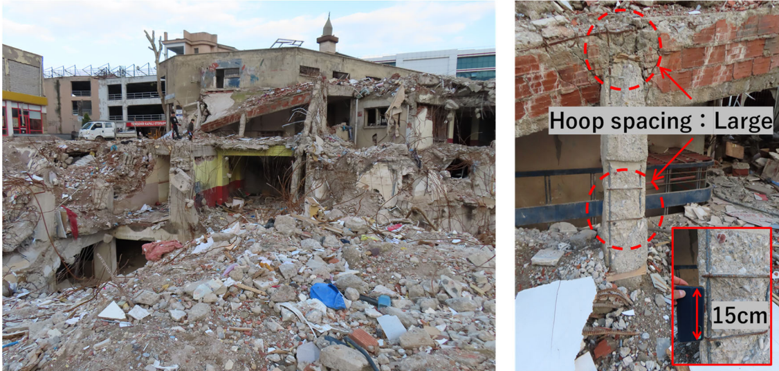
Photo 2-7 Seismic damage in Kahramanmaras (Location ⑤)
