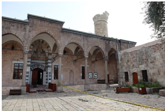
Photo 5-25 Payas, Hatay. Sokullu Mehmet Paşa Külliyesi designed by Mimar Sinan. The minaret collapsed.
