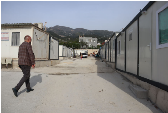
Photo 1-70 Payas, Hatay. Container temporary housing currently in use.
