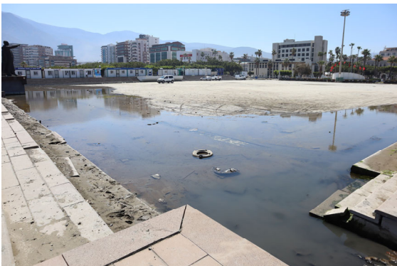
Photo 1-55 İskenderun, Hatay. Liquefaction.
