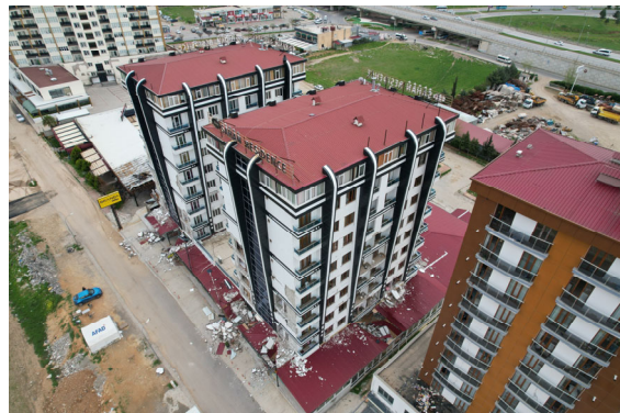
Photo 1-5 Onikişubat, K.Maraş. Drone shot of apartment buildings in Photo 1-4.
