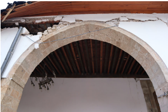
Photo 5-5 Arch section of portico
