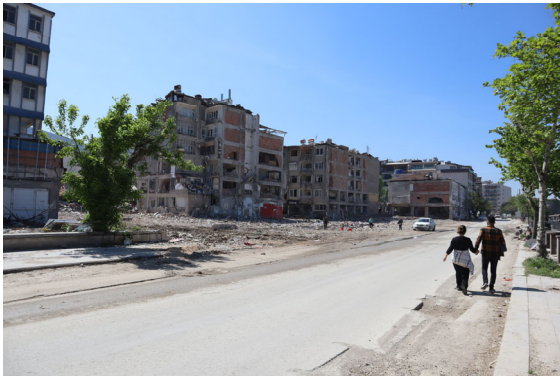
Photo 1-26 Antakya, Hatay. The seven-story townscape was gone.
