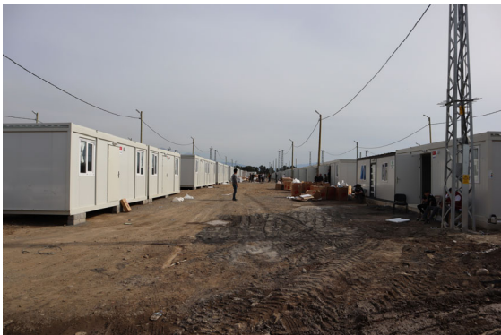
Photo 4-13 335 container temporary housing units to be completed next week. There were laundry containers, hospital containers, school containers, etc.
