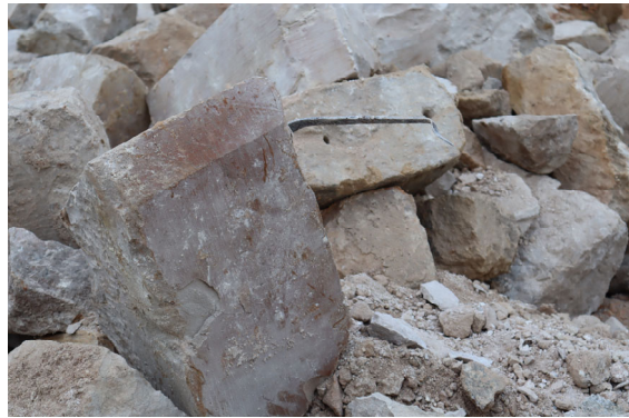
Photo 5-9 Steel tie connecting the stones of the collapsed minaret.
