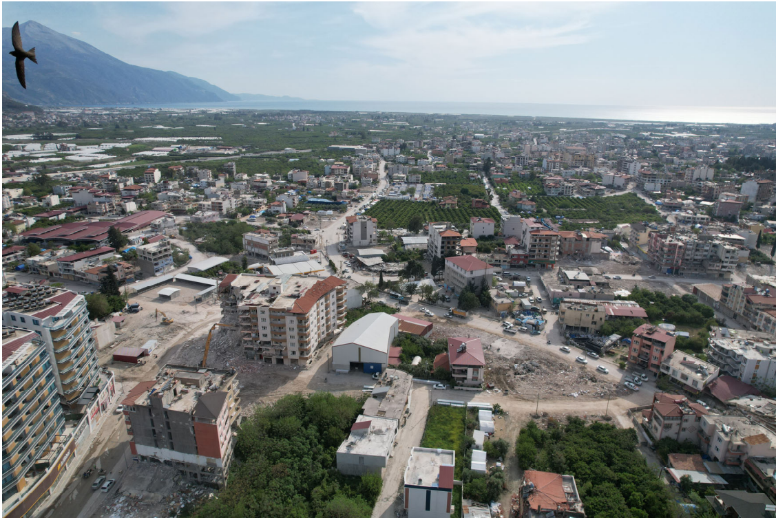
Photo 1-49 Samandağ, Hatay. Many buildings collapsed or damaged.
