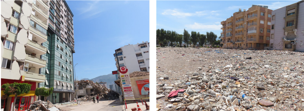
Photo 2-12 Seismic damage in Iskenderun
