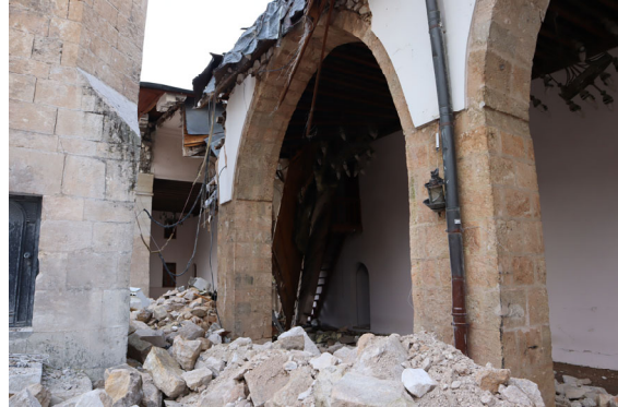
Photo 5-4 Damaged portico.
