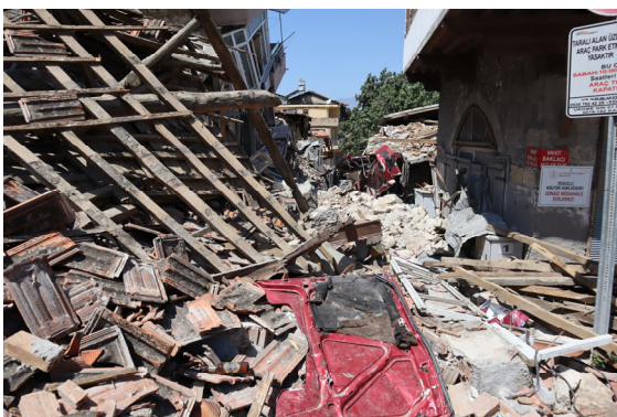
Photo 1-42 Antakya, Hatay. Alley entering from Kurtuluş Street.
