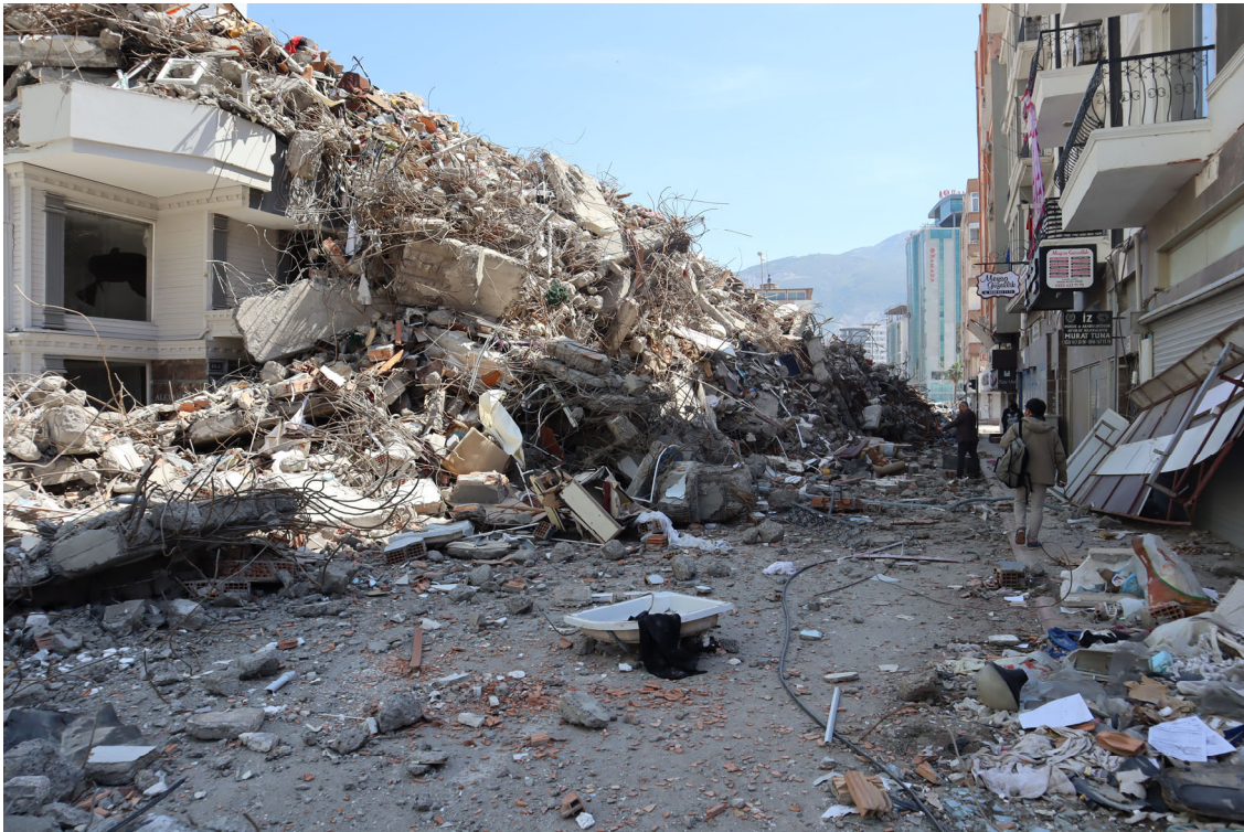
Photo 1-59 İskenderun, Hatay. Collapsed site of a 12-story apartment building.
