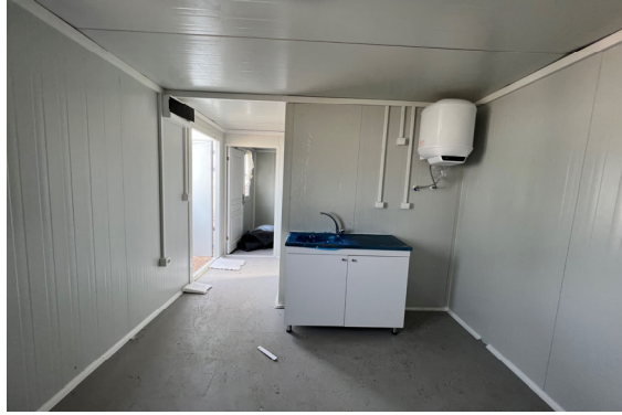
Photo 4-16 Inside the container. 21 m 2 A kitchen was attached.
