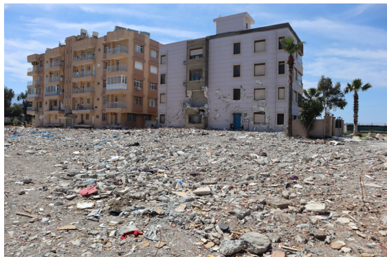
Photo 1-63 İskenderun, Hatay. A 7-story apartment building collapsed. The columns of the restaurant on the first floor had been removed by the owner.
