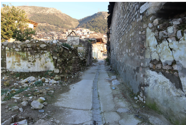
Alley spaces Have drainage channels in the middle
