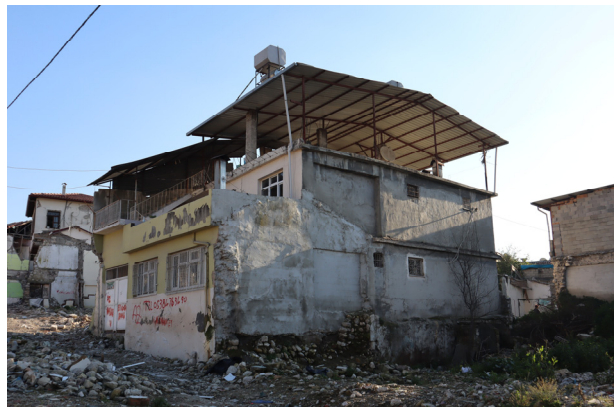
Reinforced concrete (RC) building Steel roof frame Does not suit the scenery
