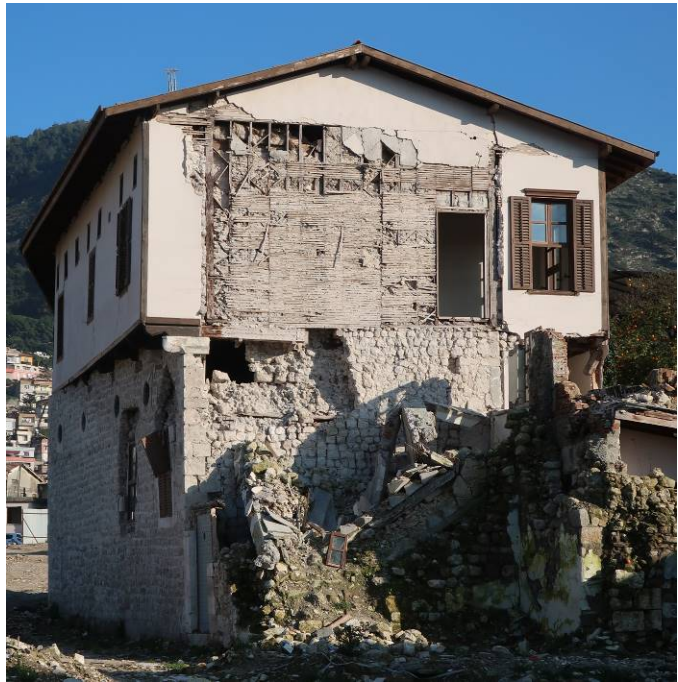
Wall of rubble stone masonry and Bağdadi wall
