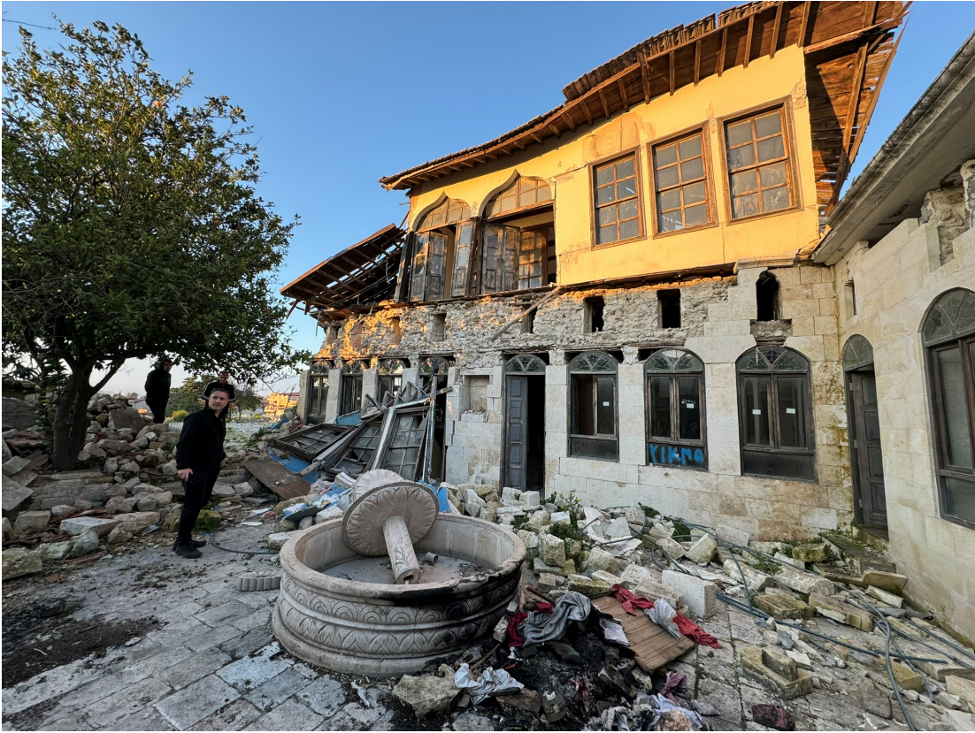
Destroyed residential building Left neglected
