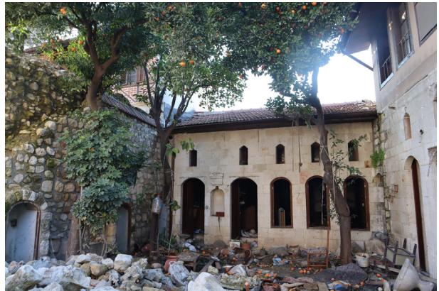
Courtyard 1st floor wall is cut stone or cobblestone 2nd floor is wooden Roof tiles are Marsilya
