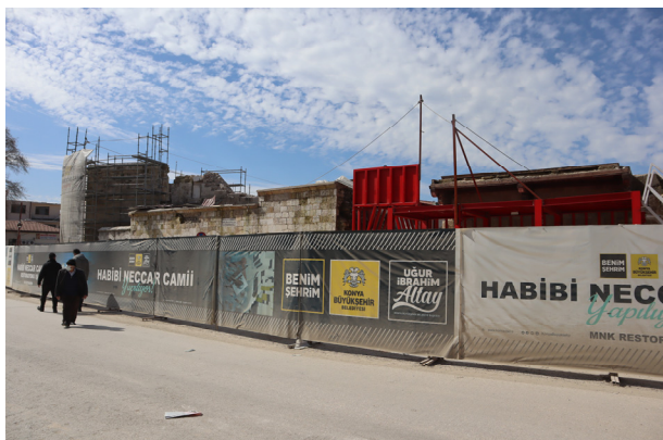
Habib-i Neccar Camii Government-initiated restoration and reconstruction underway
