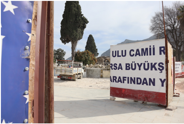
Ulu Camii Government-initiated restoration and reconstruction underway
