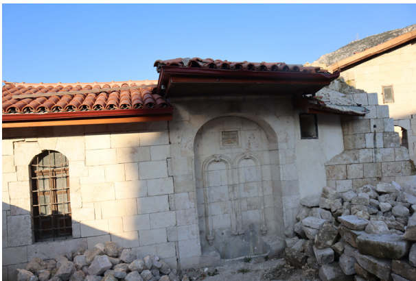
Exterior view of camii at restoration site Walls of cut stone Roof tiles are alaturca
