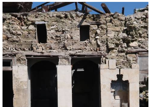
Rubble stone masonry and ashlar cladding
