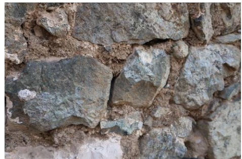
Poor mortar
