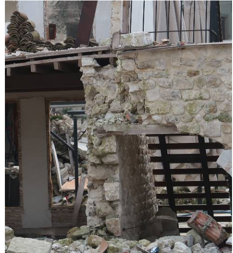
Rubble stone masonry and wooden floor
