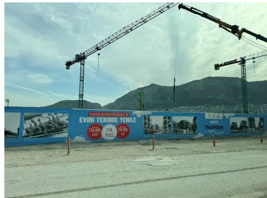
Apartment construction site along the river in the new city
