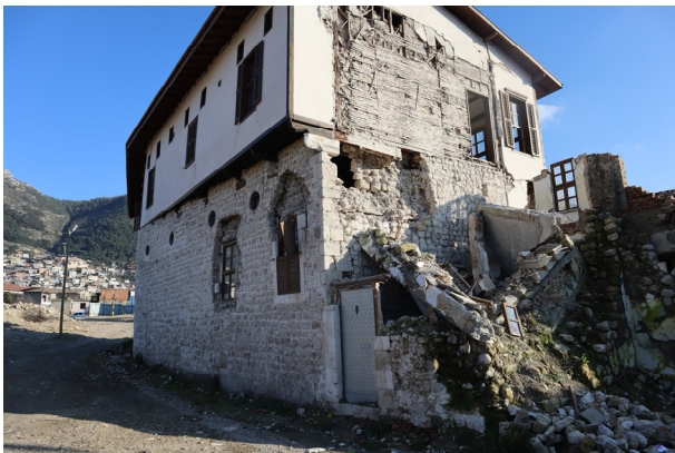
First floor made of stone Second floor made of wood Traditional construction method called bagdadi
