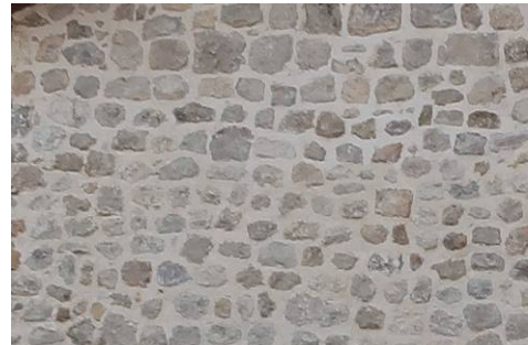
Exterior view of rubble stone masonry wall
