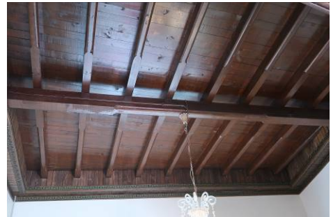
Wooden floor framing
