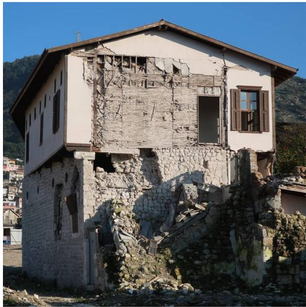
Rubble-stone masonry and Bağdadi exterior walls
