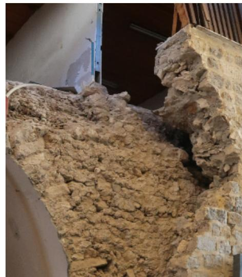
Damaged state of a rubble-stone masonry wall
