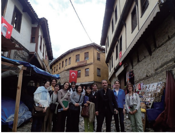
Cumalıkızık: the traditional houses feature a stone structure for the first floor and a wooden structure for the second floor.
