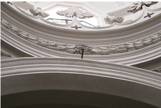
Fig 16. The dome base of the San Carlo Church. The top of the arch and the lower section of the dome base are interfering with each other. We believe this creates a spatial sense of "depth" in the relationship between moldings.
