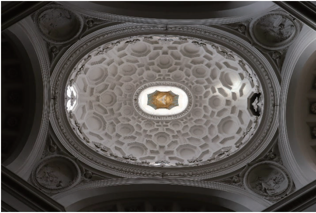
Fig 15. The dome of the San Carlo Church. It is supported by arches and pendentives. It has octagonal, hexagonal and cross coffers.
