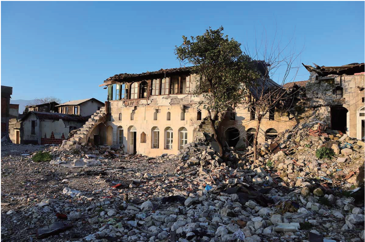
Wall surface of a house that once had a courtyard — a typical example of a residence in Antakya.
