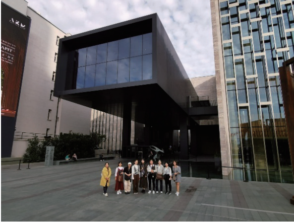
The Atatürk Cultural Center, originally opened in the 1960s, has recently reopened after technical restoration that preserved the original design by architect Murat Tabanlıoğlu, son of Hayati Tabanlıoğlu, the original design architect.
