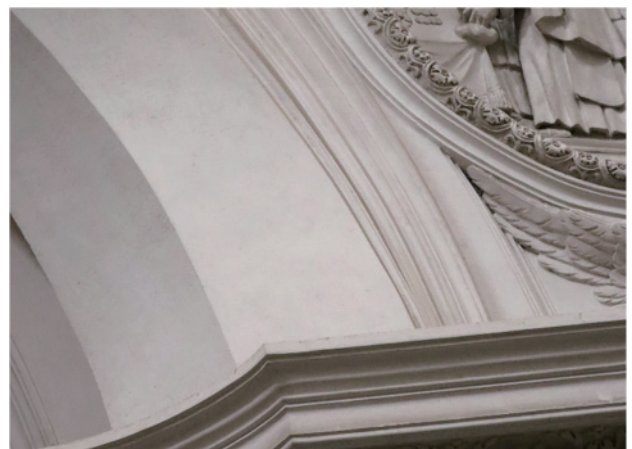
Fig 13. Bottom of the semi-oval arch. The intrados squeezes the moldings, giving them a cramped appearance. The smooth surface shrinks from the top to the bottom of the arch, changing the configuration to one in which the moldings are densely packed.
