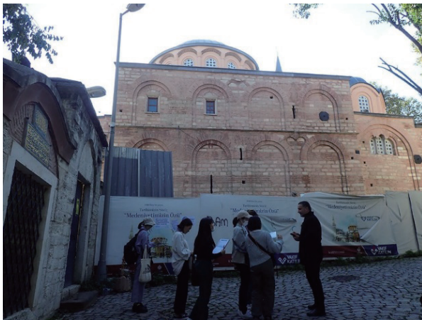
The Kariye Mosque recently underwent renovation.
