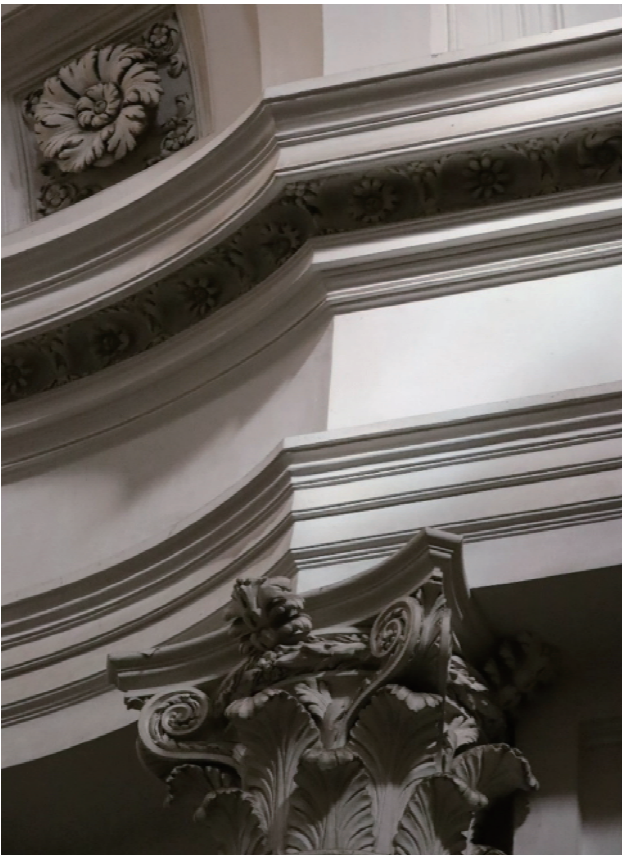
Fig 4. The entablature of the San Carlo Church, comprising of “architrave,” “frieze” and “cornice”. Although there is no relief decoration, rich shadows and light coexist. The cornice has particularly dark shadows, and the frieze glows white.
