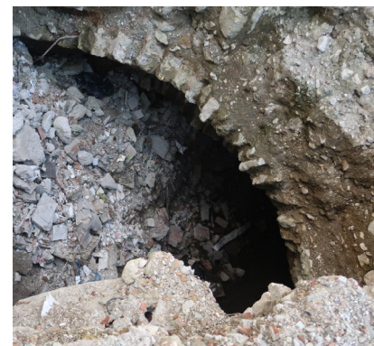
Exposed Roman culvert
